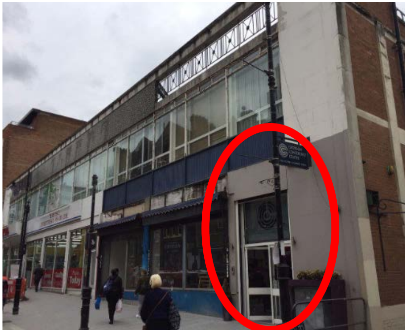
Croydon Conference Centre
